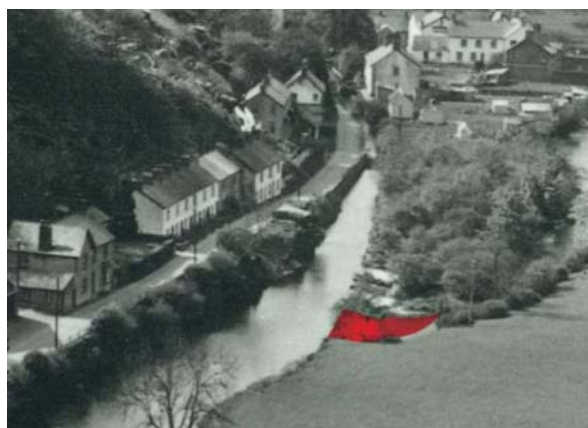
Photo 4: A 1930's photograph the red shaded area showing weir that is now part of the river bank
