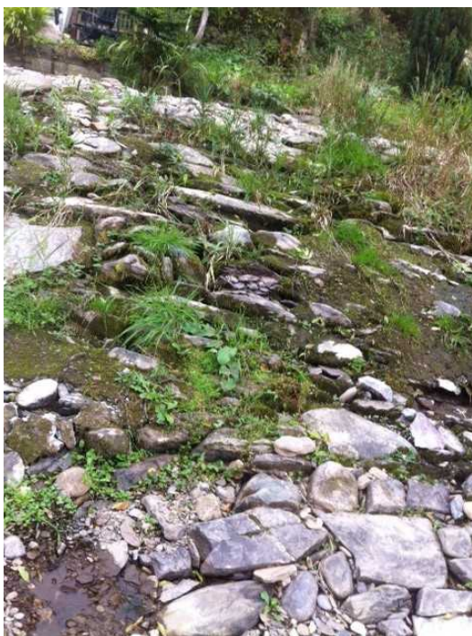
Photo 1: Dulverton Weir section showing original rounded stones still in position
